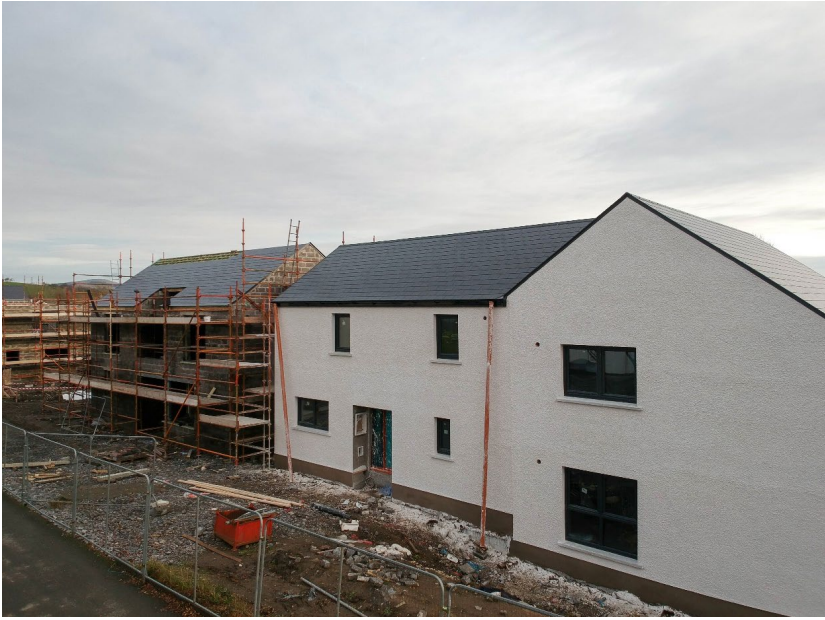
Photo 1: Railway Park, Donegal Town (Phase III)
