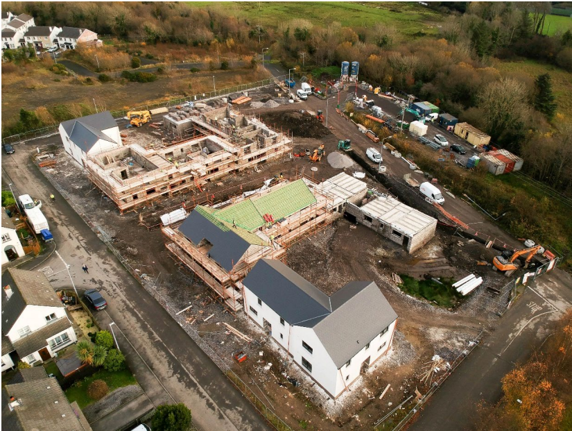
Photo 2: Railway Park, Donegal Town (Phase III)
